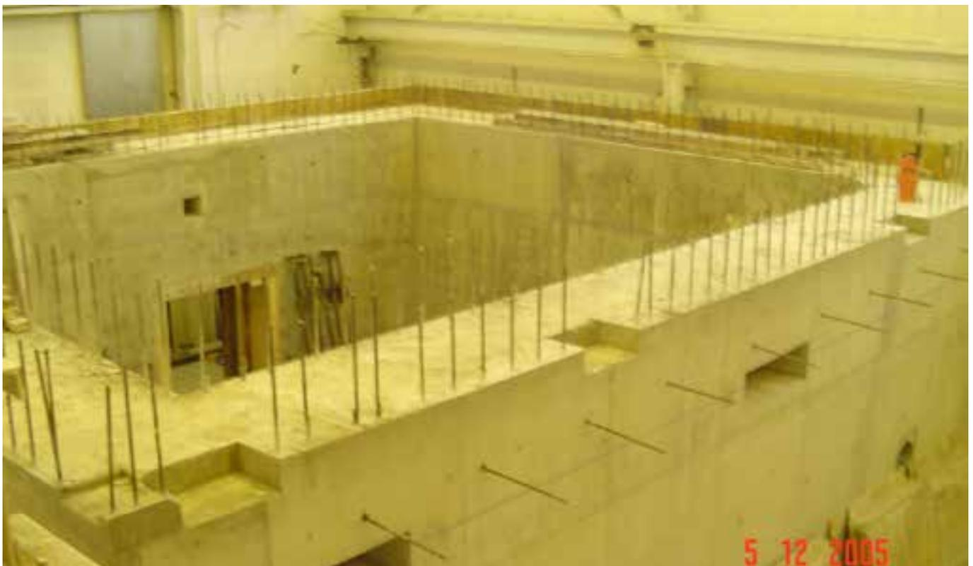
*Target Area 3 bunker from the south east corner showing the metre-thick concrete walls, December 2005. The roof of TA3/floor of LA3 has yet to be added so you can see the entrance door to the bunker.*
