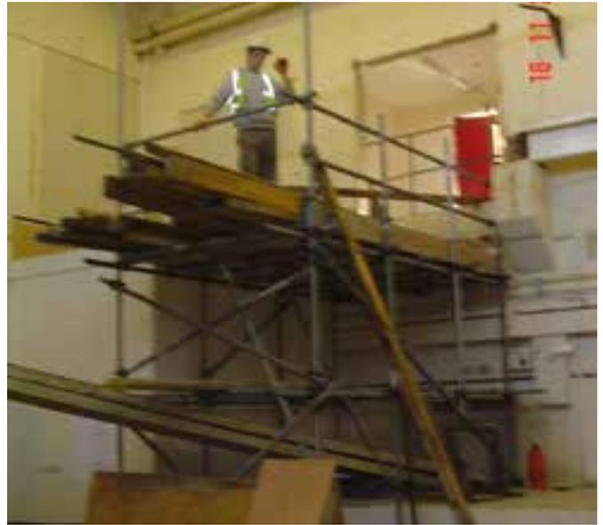
*Build-up of shuttering for the TA3 bunker. The doorway hanging in mid-air is the door into Laser Area 3.*
