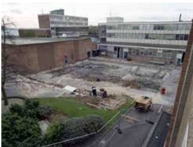
Ground work begins outside R1, digging up what used to be the Director's car park. The new building was approximately 21.5m x 24.5m in size, consisting of a brick faced external skin, 30 cm thick concrete radiation shielding walls, and an aluminium skin roof.
