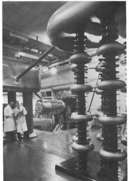
The Cockcroft - Walton high voltage generator with the injector of the proton - linear accelerator in the centre - background.
