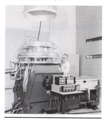
Attaching accelerometers to the RAL liquid helium cryostat on the electromagnetic vibrator, before vibration-testing the Long Wavelength Spectrometer at 4K. The spectrometer will be one of the instruments on board the Infrared Space Observatory to be launched by ESA in 1993.
