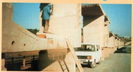
Structural monitoring devices are built into Bideford Bridge during construction. (Photo: Bristol University)
