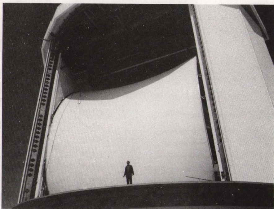
The Telescope enclosure showing the membrane installation.
