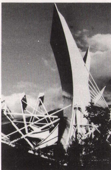
The antenna for the new EISCAT VHF system at Tromso: the huge parabolic cylinder reflector has total dimensions of 120 by 40 metres.
