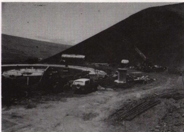
This general view of the site shows the central telescope foundation, to the left, with the Carousel foundation ring beam around.
