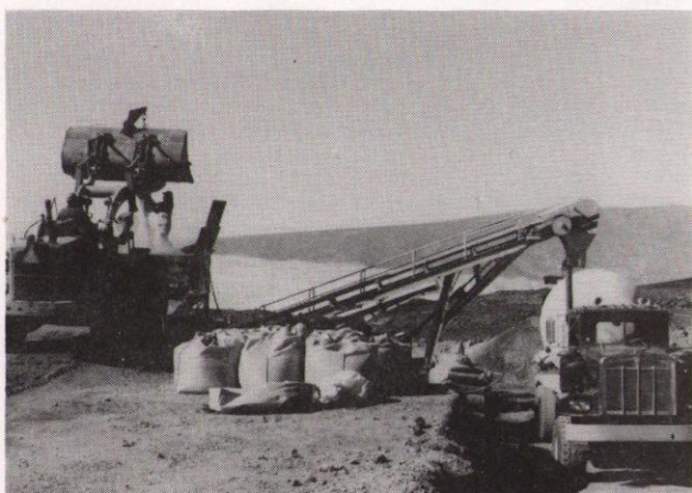
The concrete batching plant above the clouds at 3660m altitude.
