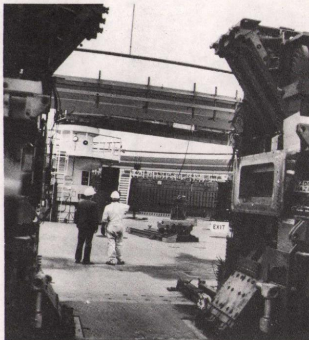
An accelerating cavity has been removed from Nimrod's main ring of magnets to allow trucks to enter.
