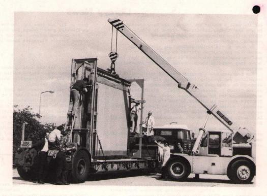
There was intense activity near building R12 at the end of August, as all hands were put to the task of loading an enormous drift chamber onto a flat-bed trailer. This is the first of a series of drift chambers, built at the Rutherford Laboratory, for use in the European Muon Collaboration experiments at the CERN Super Proton Synchrotron (SPS) in Geneva, Switzerland.
