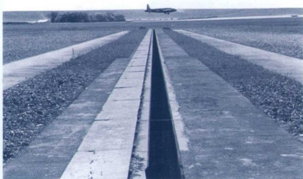
Catapult trench showing slot for travelling hook. Tracks for Avro Manchester bomber undercarriage are on either side. In the distance a Wellington bomber is landing.
