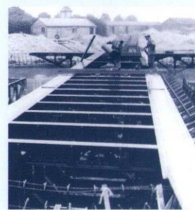
Construction of turntable roof section.
