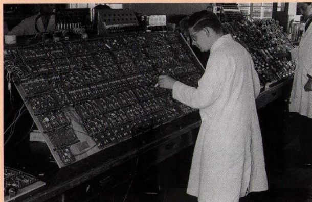
Jim Stevens circuit testing the world's first transistorised computer, built by Electronics Division in 1958. (A 3733)
