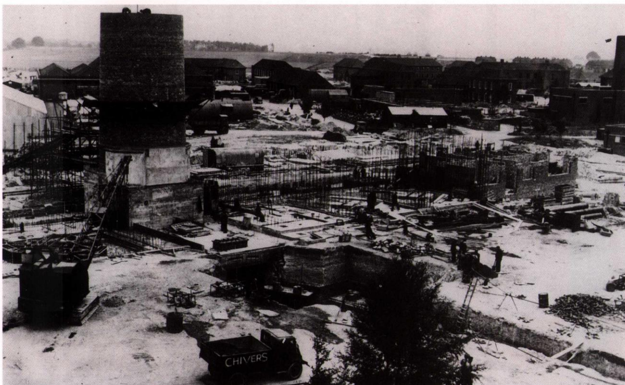
Work starts on the BEPO stack in November 1947. The Ministry of Works architects originally specified an eight-sided design, but a circular one was built for expediency. In the foreground can be seen the main air-duct for BEPO. The RAF's boiler house (top right) was demolished to make way for building 424. (HR 101572)
