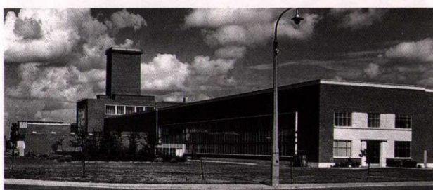
The Radiochemistry Laboratory B220, was completed in mid 1949 to a unique specification; air conditioning plant in the windowless upper storey cleans the entire volume of air in the building twice a second. One wing is used for alpha-emitting materials, the other for beta/gamma work. Internal walls are made with rounded corners to avoid trapping dust particles and coated with strippable rubber paint to aid decontamination. Light fittings were recessed, windows hermetically sealed and the interior finished off to a hospital standard. Doors opened and closed automatically. (HPC 84853)
