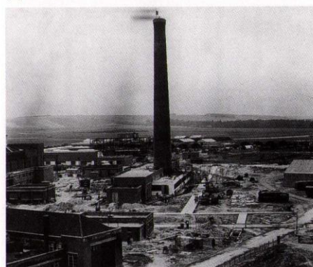
The "topping out" of BEPO's 200ft stack in 1948. BEPO required five tons of air every hour to limit the uranium fuel temperature to below 200 degrees Centigrade. The air exhausting from the stack pierced the densest fog. (HR 59797)
