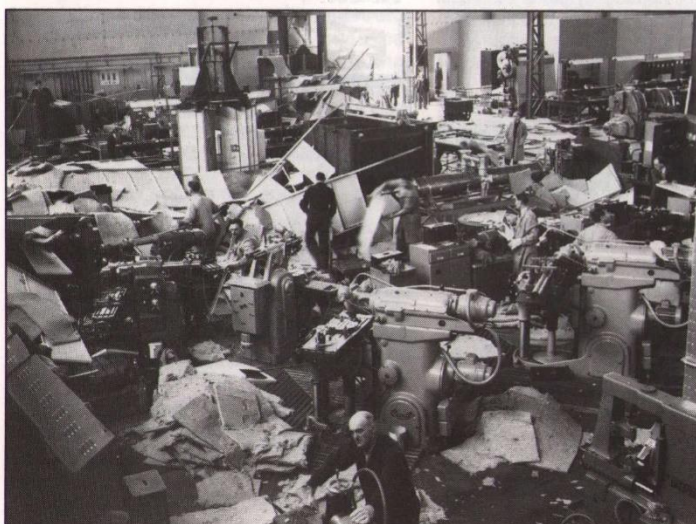
A suspended ceiling of perforated metal tiles with an insulated backing had been fitted in an attempt to cut down the heating bill for Hangar 9 — it nearly cut down the workforce instead when, one day in 1959, it collapsed and they all had to dive for cover!
