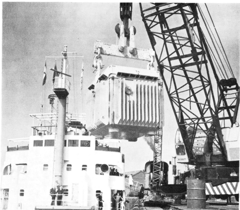
The Leven Fisher, chartered by the United Kingdom Atomic Energy Authority from James Fisher and Sons Ltd. of Barrow, is seen at Whitehaven docks unloading a consignment of irradiated fuel from the Tokai-mura reactor in Japan.
