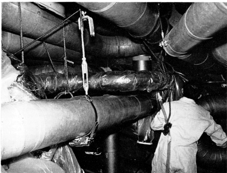
The section of repaired pipe (in polythene wrapping) being replaced preparatory to welding.
