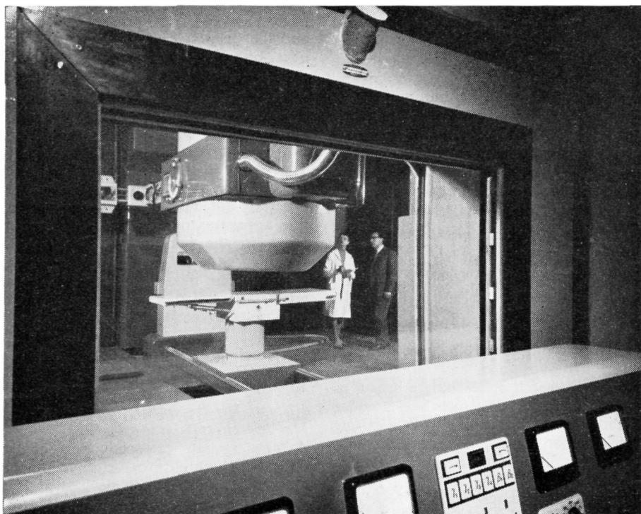
A three foot thick Harwell type zinc bromide viewing window used in the Betatron cancer unit at St. Luke's Hospital, Guildford.
