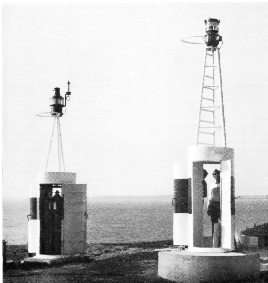
The first British isotope-powered marine light to be used abroad (right) is installed on the west coast of Sjaeland, alongside the existing acetylene lamp.
