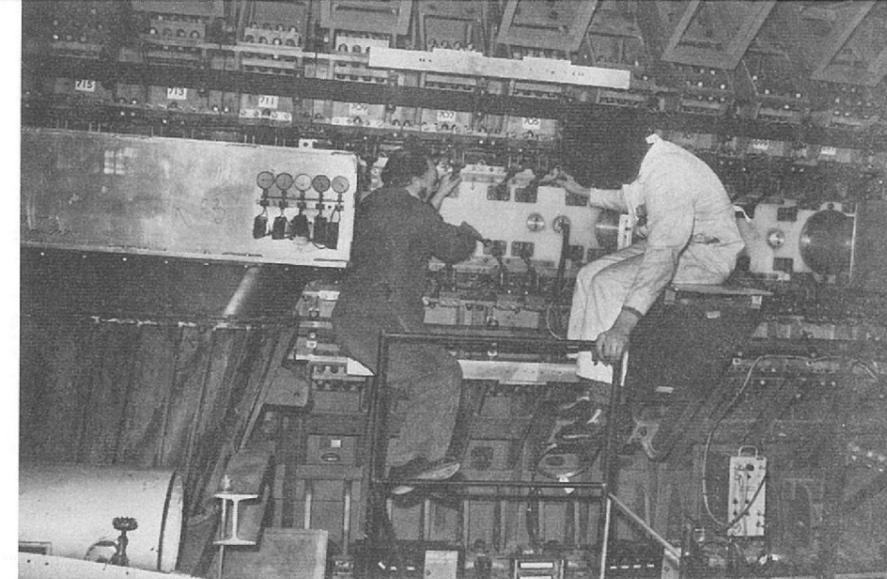
Figure 64. Fitting a new polythene closure plate to the vacuum tank of Nimrod (see opposite) : (12511).
