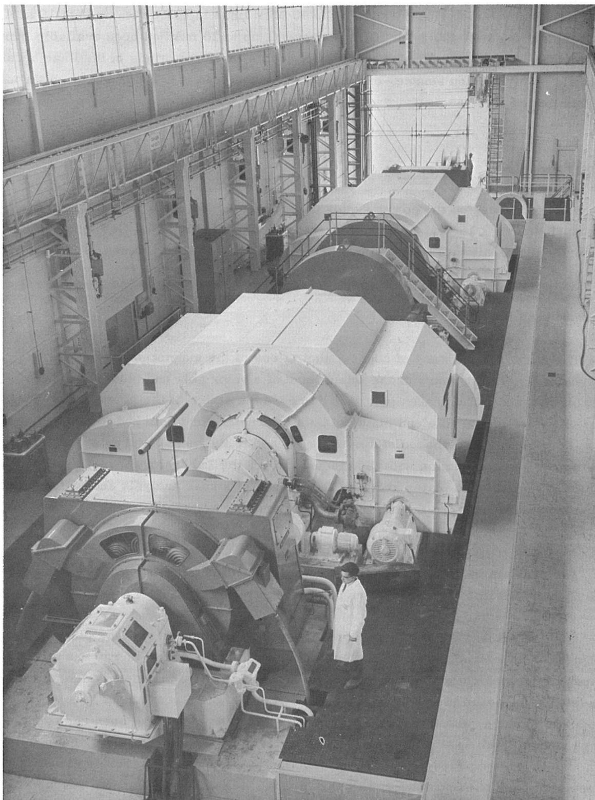
Figure 21. The Nimrod main magnet power supply alternator set.
