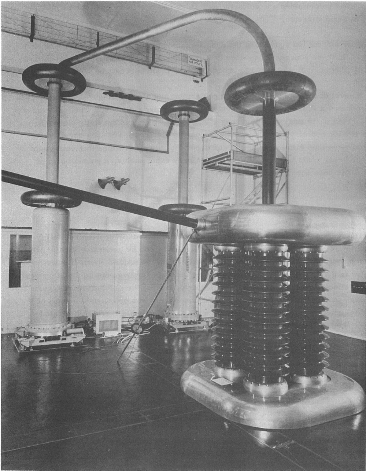
Figure 23. The two 600 kV generators for the preinjector are shown in the background with the new type of termination. Rapid changeover of generators is achieved by swinging the top arm from one to the other.
