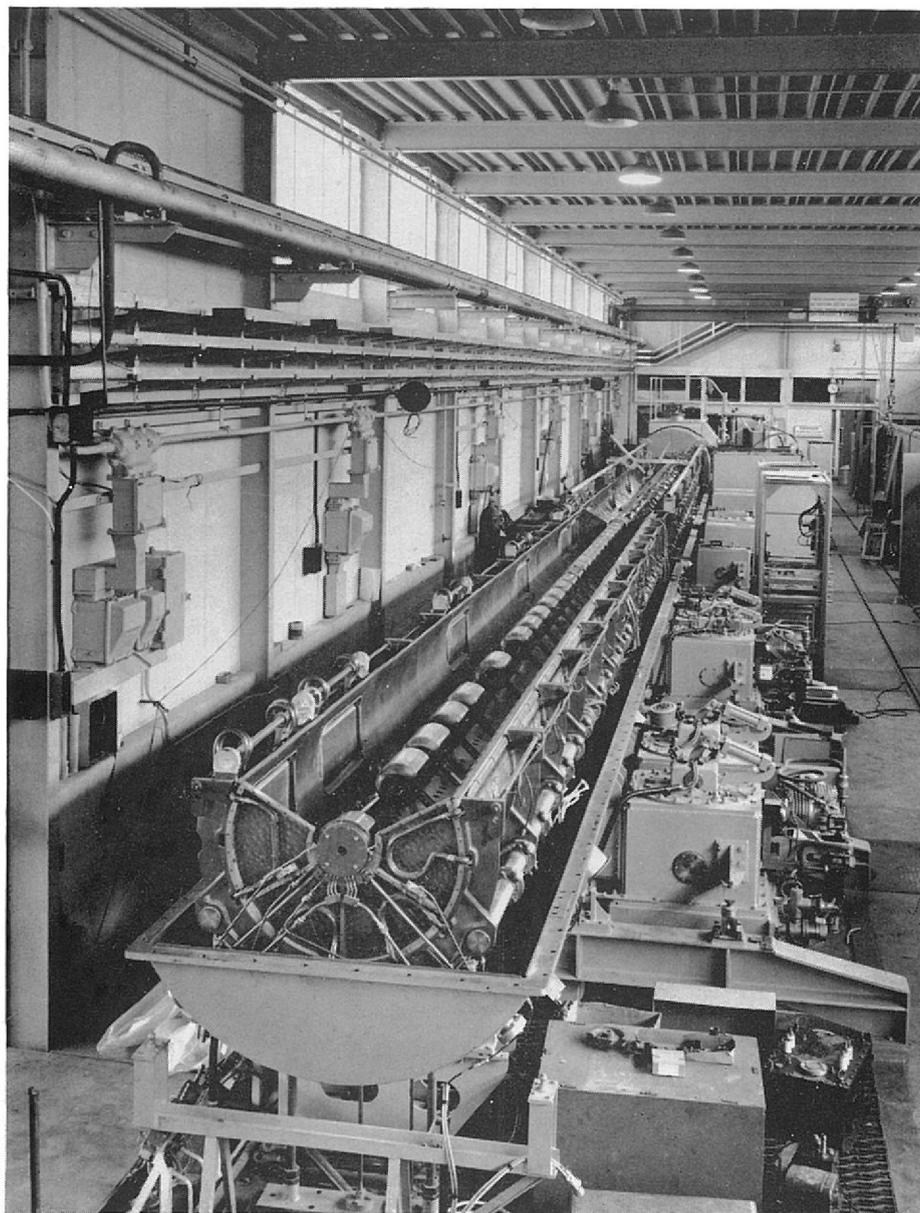
Exposed view of drift tubes in tank III of the 50 MeV Proton Linear Accelerator
