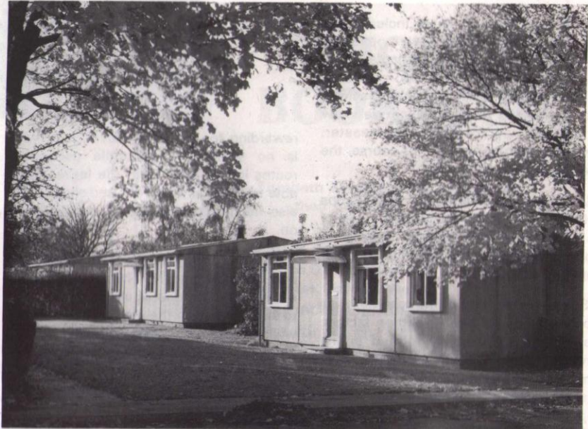
MOW prefabs on the Authority estate at Chilton
