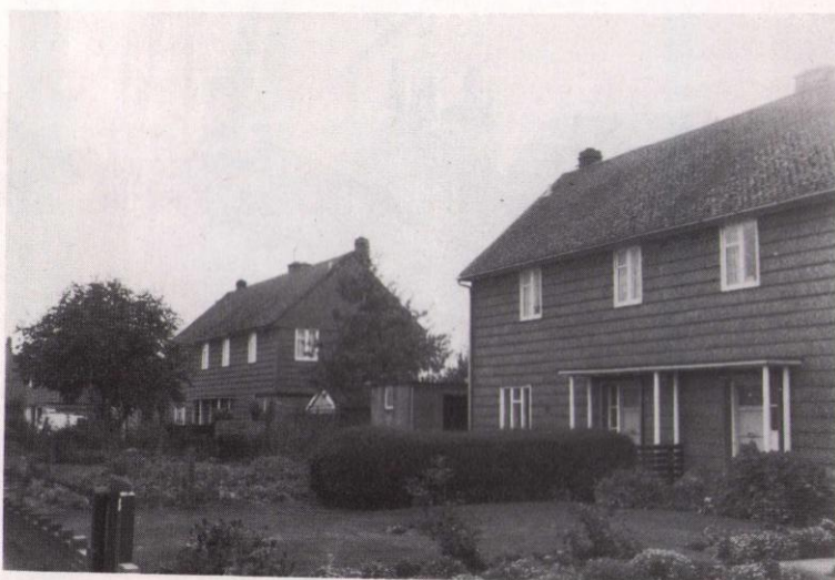
An "Airey" house at East Hagbourne
