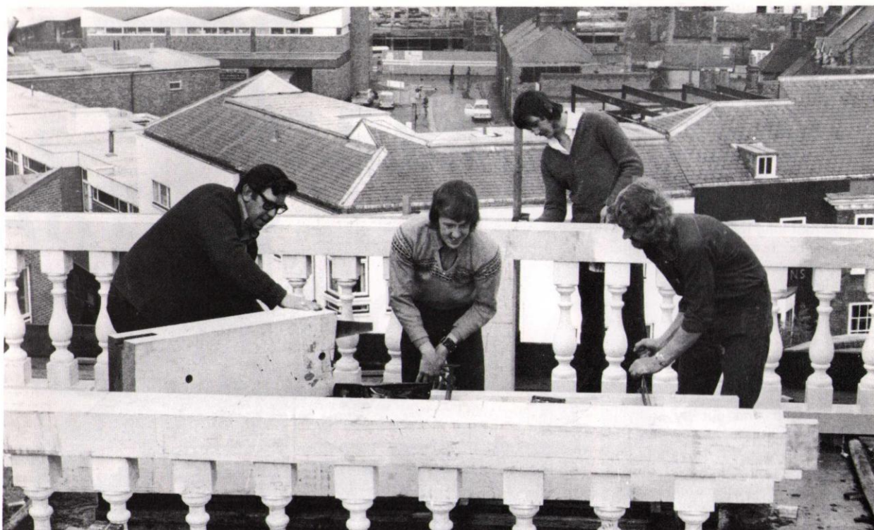
Work in hand renovating the balustrade of County Hall
