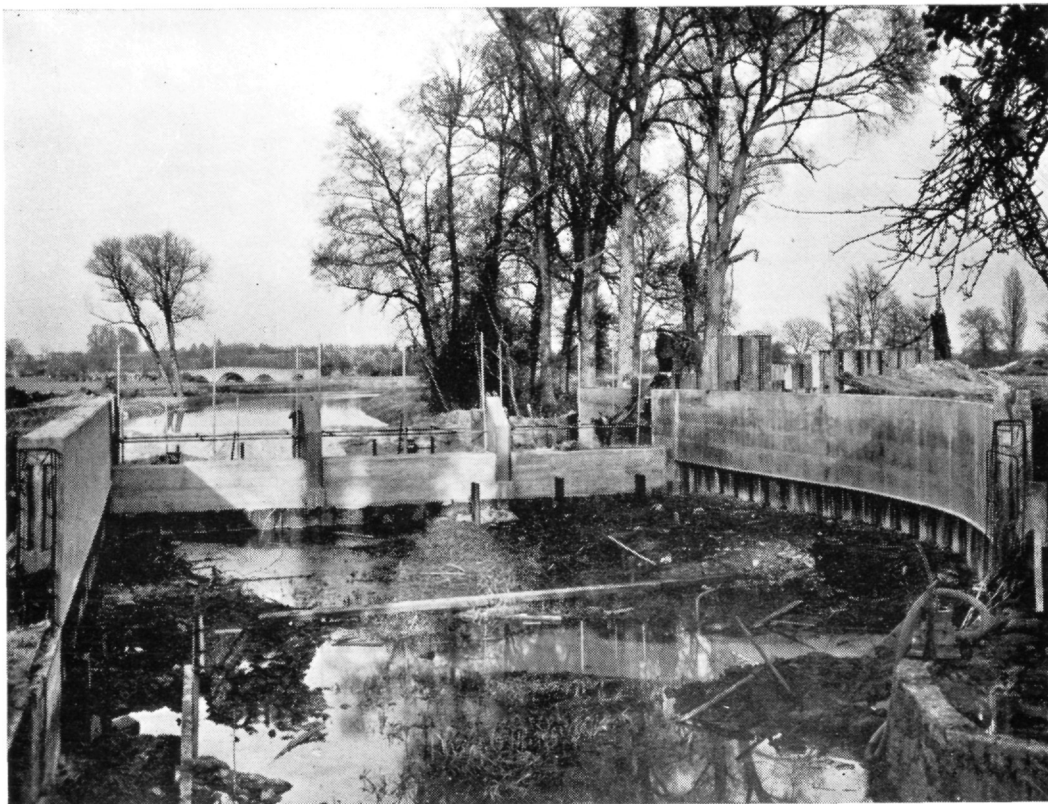
Construction of weir for effluent outfall at Sutton Courtenay, Feb. 1948
