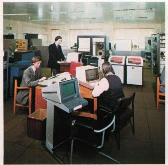
Work in progress at Chilton to assess the comparative performance of two minicomputers for interactive use. On the left is a GEC 4070; background centre is a Prime 400. Local terminals (foreground) include a thermal printer, alphanumeric VDU and storage-screen devices.
