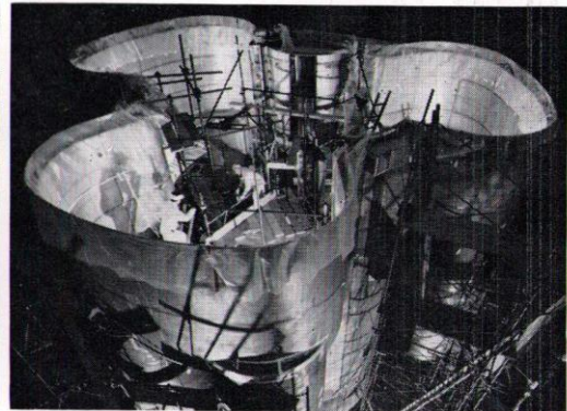
Prototype fast Reactor at Dounreay
