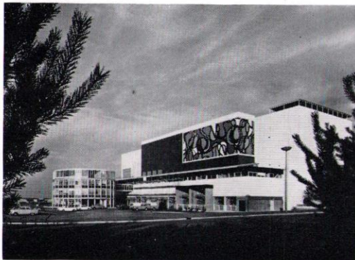
SGHW Reactor at AEE Winfrith
