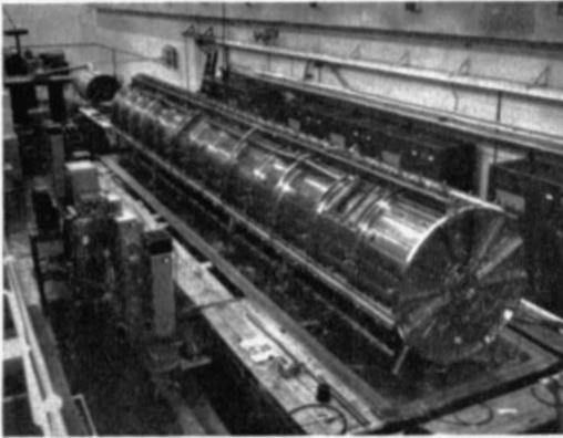
Figure 2. 15 mev injector for NIMROD, under construction.
