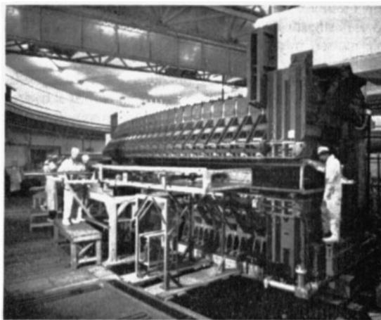
Figure 5. Installation of NIMROD inner vacuum vessel.
