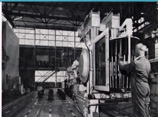
Calder Hall reactor charging floor showing fuel elements and a charge machine.
